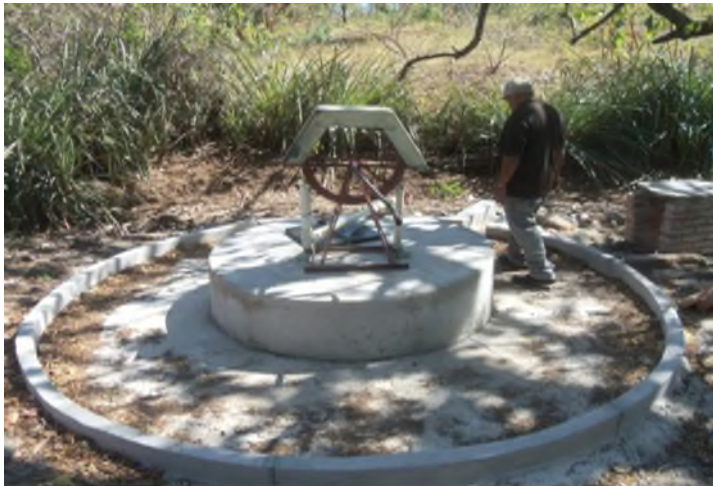
Construction of small community water storage facilities
