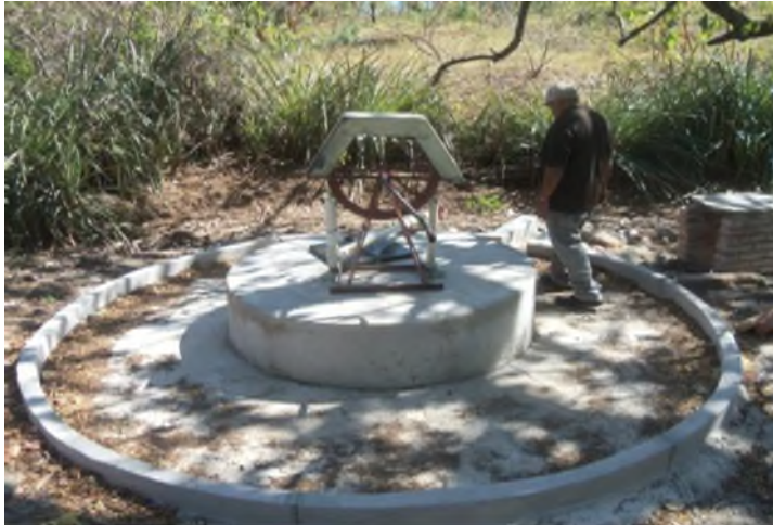
Construction of small community water storage facilities
